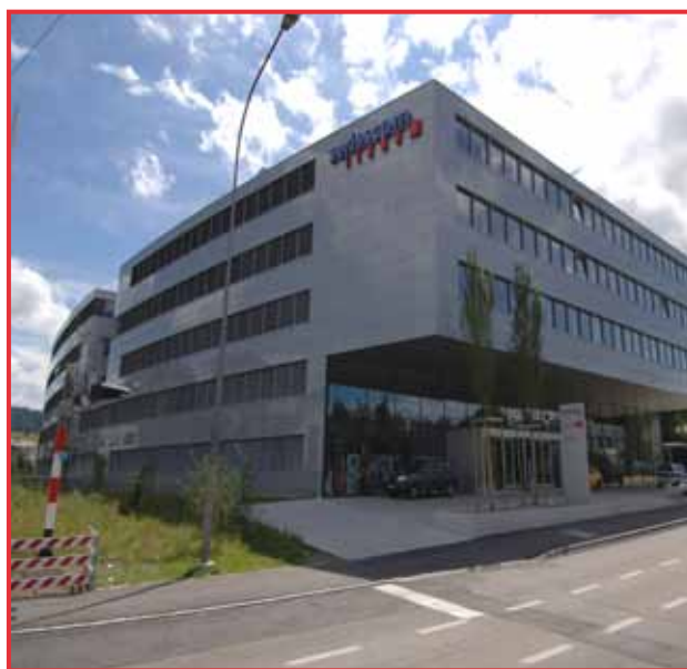
Nouvelle construction Business Park, Liebfeld, BE-575
